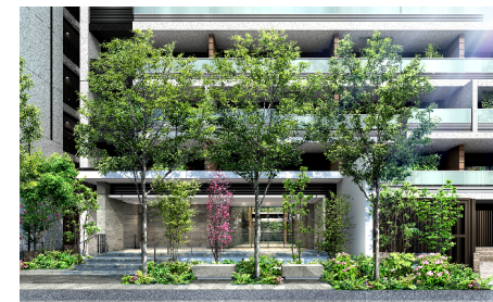
CLIO RESIDENCE YOKOHAMA TSUNASHIMA (provided in 2020)
