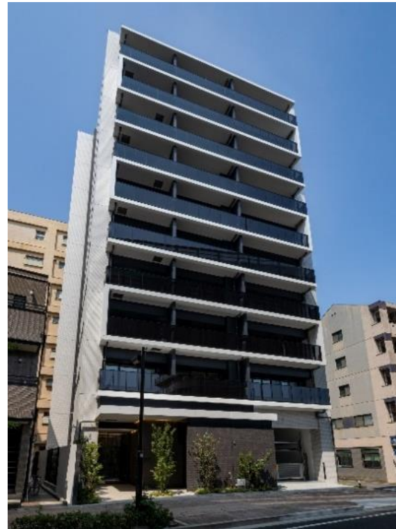
Nagoya, Aichi Total number of units: 28 Delivered in September 2022
